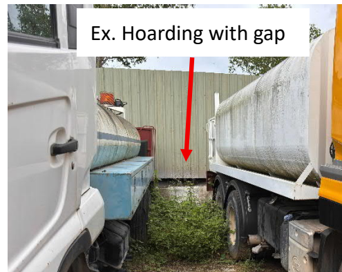
Photo 12 – Ex. Hoarding with gap along southern boundary
