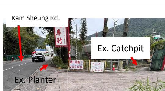
Photo 7 – Existing Planter & Catchpit
