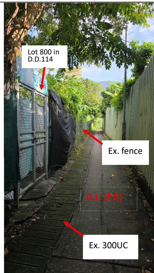
Photo 16 – Ex. Ditch outside southern boundary
