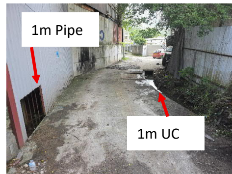
Photo 4 - Downstream Facilities (1m Pipe & 1m UC)
