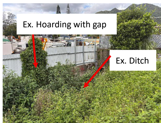
Photo 13 – Ex. Hoarding with gap along southern boundary
